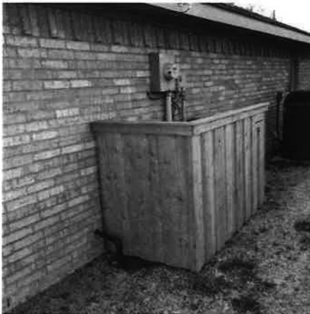
a Cart Bin Storage
